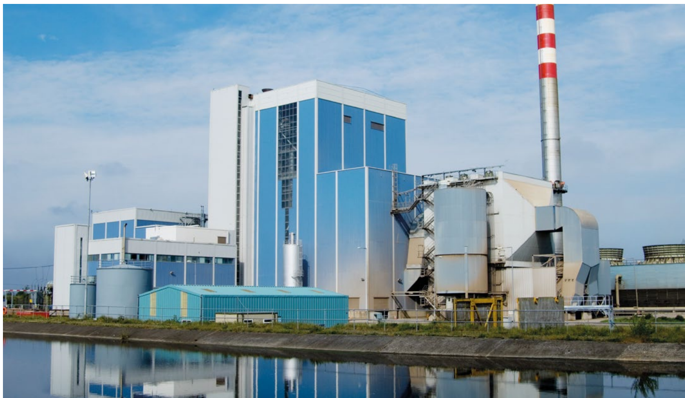
Edenderry Power Plant.
